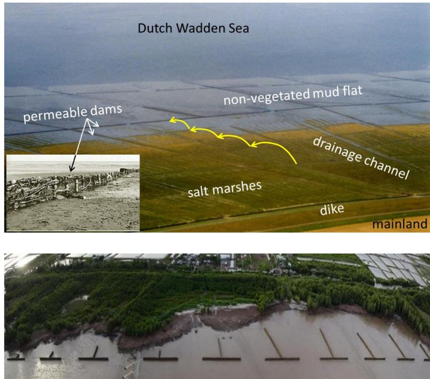
Figure 7.1 Sedimentation basins constructed by permeable structures in the Wadden Sea, The Netherlands (above) and in Vietnam (below).
