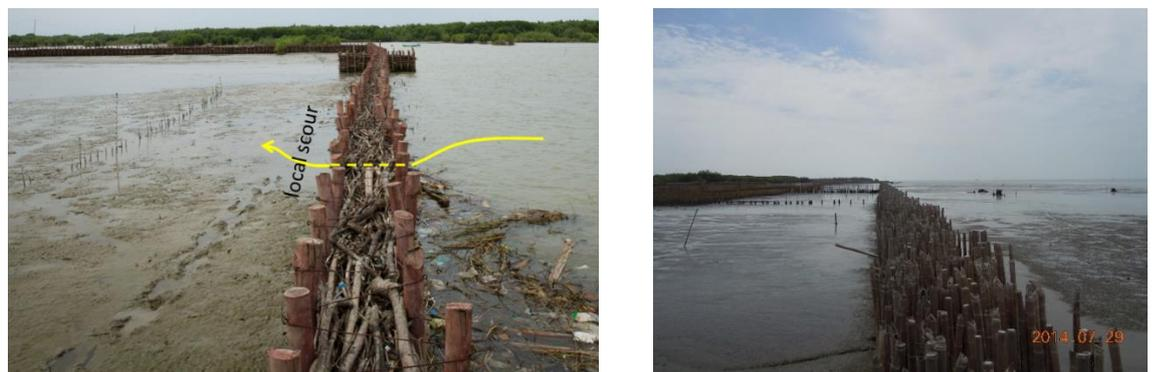
Figure 7.2 Left panel: “classical” permeable structure with brushwood; right panel: bamboo fence (both deployments in Indonesia)
