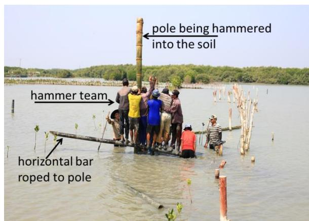
Figure 16.2 Hammer team at work to place bamboo pole, Bogorame, Demak, Indonesia.
